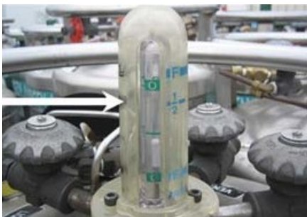
Figure 3: Older Style Sight Gauge (Typical)
